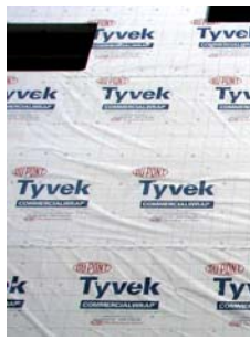
Signs of an Air Barrier issue. Not Properly Sealed.
