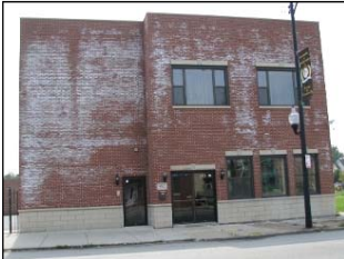
Signs of an Air Barrier issue. Not Properly Sealed.
