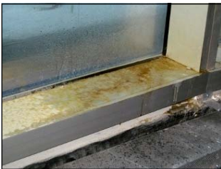
Signs of an Air Barrier issue. Dirty condensation water
